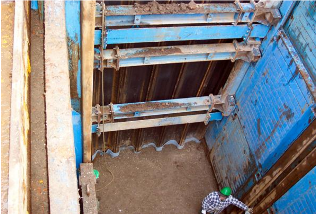
↑ Head shoring with sheet piles
