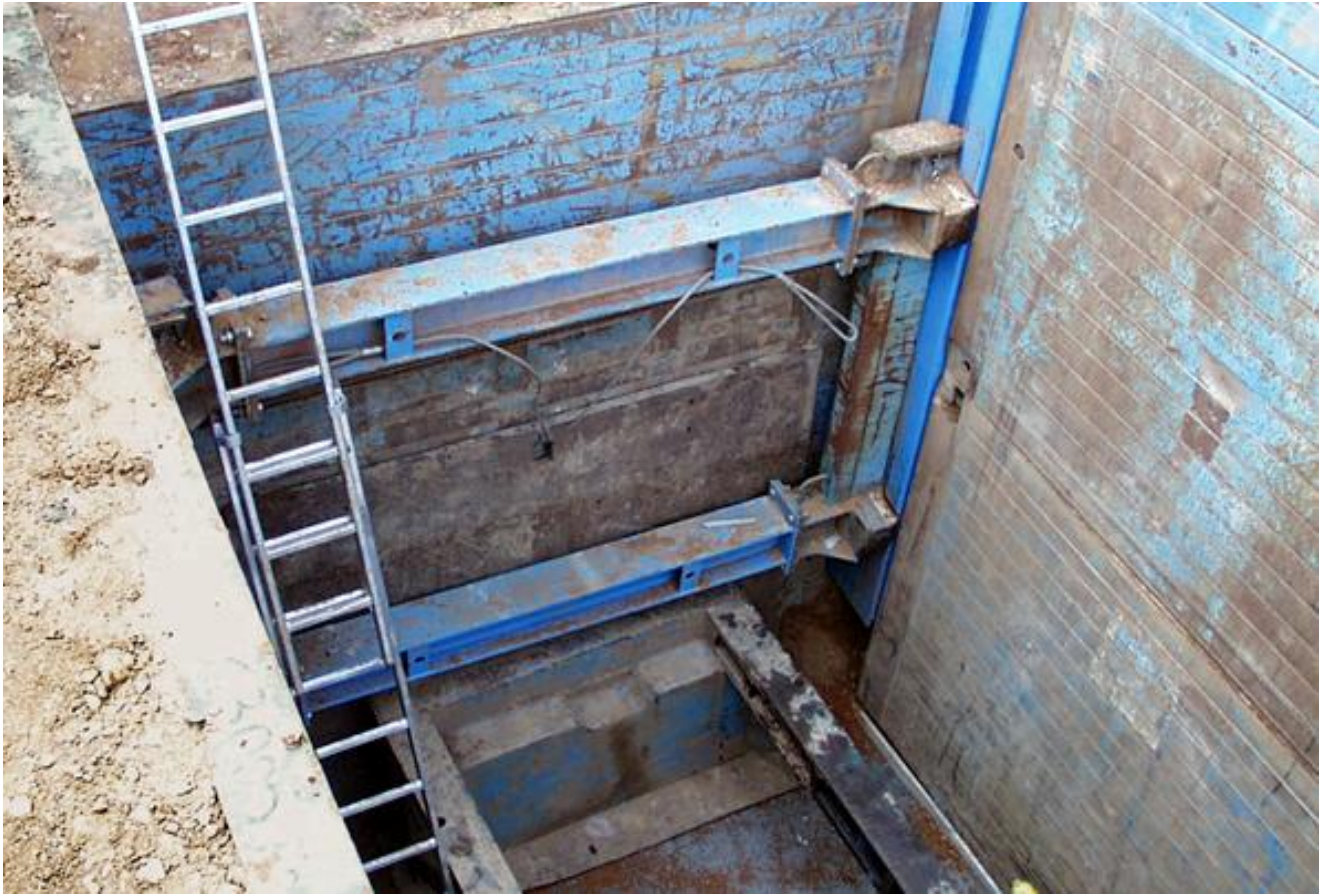
↑ Trench end shoring with single slide rail system
